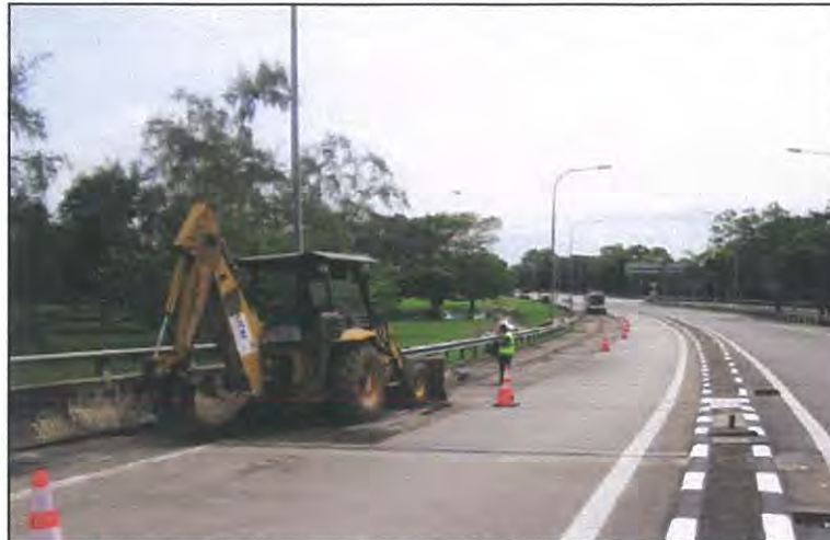
Figure 3. Milling process to scrape-off the existing asphalt layers
