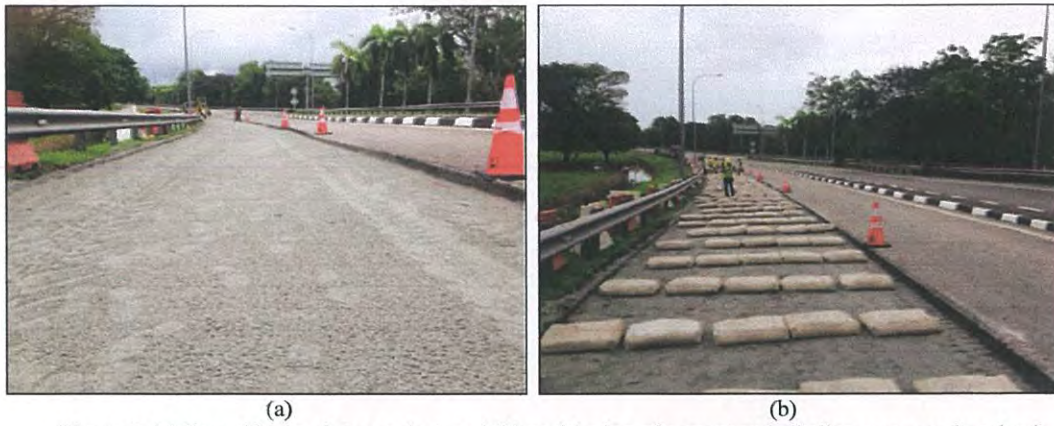
Figure 4. (a) Spread layer of quarry dust; and (b) positioning of cement and alkaline compound packaging to ensure an evenly distribution over the stabilized area
