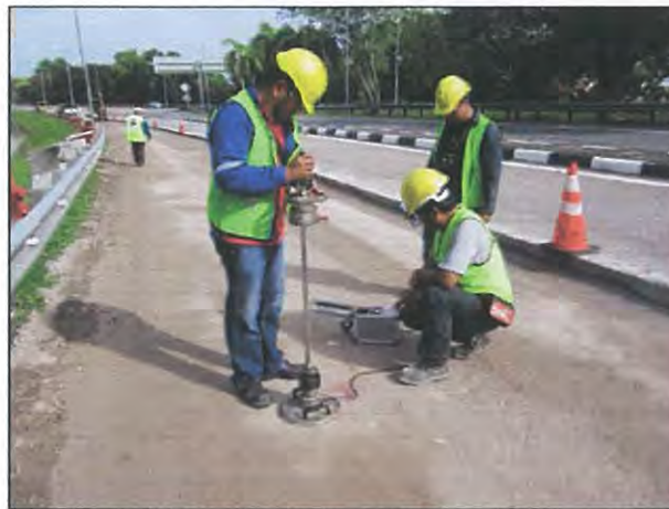
Figure 7. In-situ practical of Light Falling Weight Deflectometer (LFWD) test
