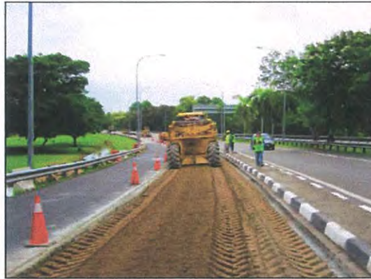
Figure 5. Mixing process of mixed soil-OPC-alkaline compound by special rotary mixer machine, CAT RM500
