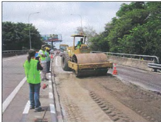
Figure 6. Compaction process by a 10 tonnes drum roller without and with vibration
